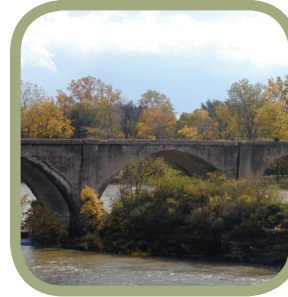
Former interurban bridge
